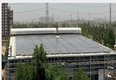
Solar panels at Bhiwadi site
